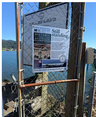
The Boathouse approach on Bay Lane is obscured with fencing and poor sight-lines.
