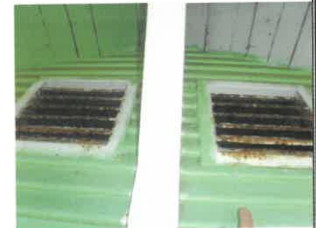
Gable end vent screens need replacement.
