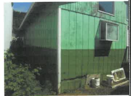
Siding has deterioration mostly at the South.
