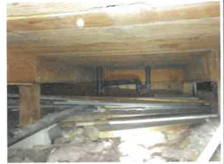
Plumbing lines under the bathroom were in satisfactory condition at the time of inspection (crawl space view).
