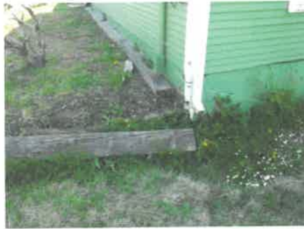
Recommend adding 6-8 foot downspout extensions to divert runoff away from the structure.
