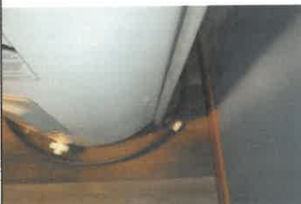
Water heater is equipped with a drip pan. Pan does not drain to the exterior. Monitor for moisture buildup.
