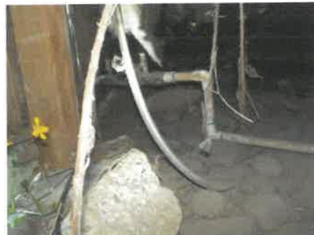
Water shutoff valve is located in the crawlspace inside the access panel.
