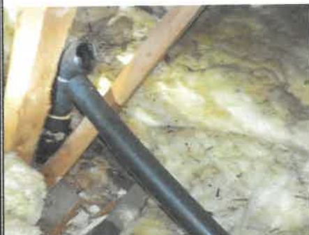
Plumbing vent lines (attic) need repair.
