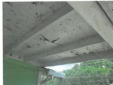
Supports and several pieces of decking have deterioration.
