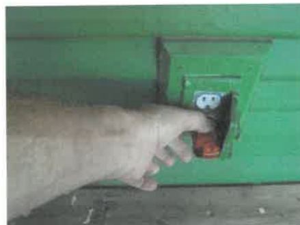
Exterior outlet isn't GFCI protected.
