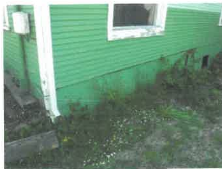
Skirting has deterioration. Openings in the skirting will allow pests to intrude.
