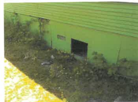
Skirting has ground contact in several areas causing deterioration.
