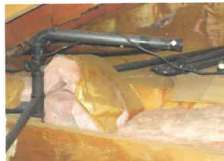
Plumbing vent in the attic wasn't extended to the exterior.
