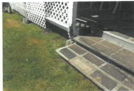
Supports and several pieces of decking have deterioration.
