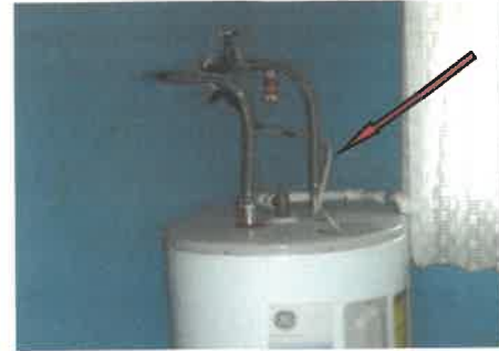
Electrical is exposed and should be protected in conduit.
