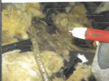
An unprotected electrical line was found in the crawlspace. Line isn't live. Removal is recommended.
