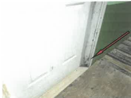
Rear entrance door has deterioration/damage to the frame and door.
