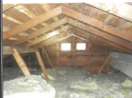
Gable end vent screens need replacing.
