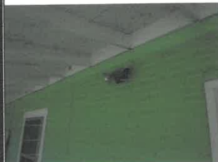
Motion detector light at the main entrance needs replacement.
