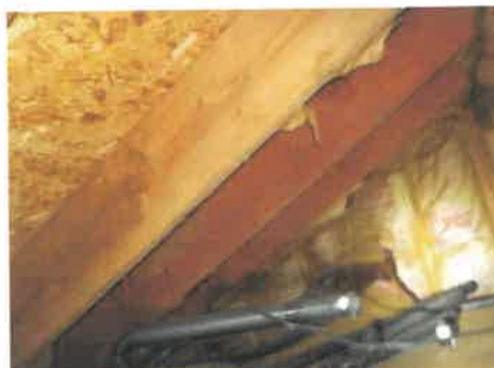
2x12 rafters are visible at the new construction section.
