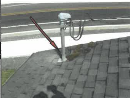
Service drop mast is sealed with mastic. Recommend using a rubber seal.
