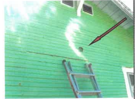
Live electrical was found in an open junction box (exterior) at the North gable.
