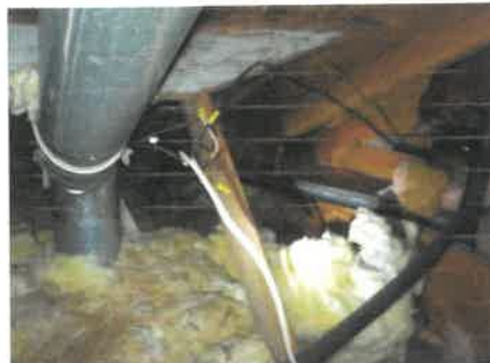
Exposed electrical connection (attic) should be in a junction box.
